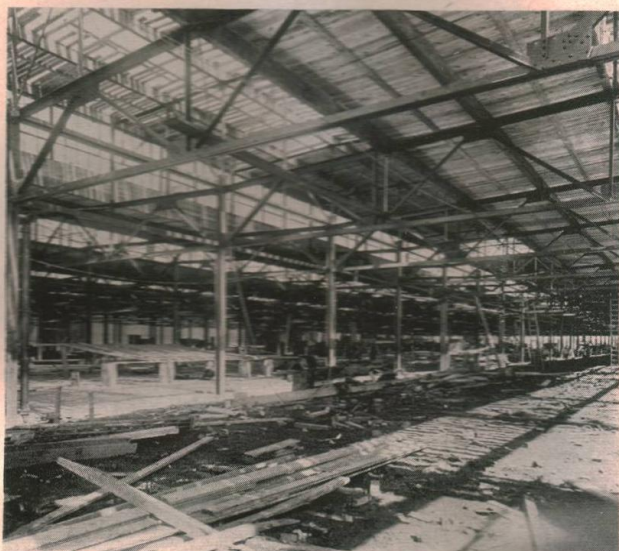
World's largest airplane plant was built at North Elmwood, Buffalo, for Curtiss. It covered 72 acres, was finished in three months, produced mostly Curtiss "Jenny" trainers. Picture looks exactly like dozens of construction shots being published today.
