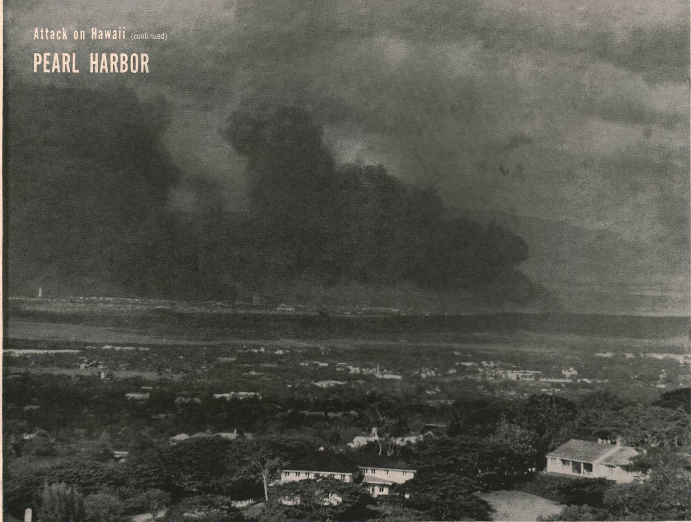
The smoke of disaster spreads thick over the island of Oahu. You are looking west toward Pearl Harbor ten miles away. Its channel to the Pacific runs off to the left. The remote white ob-
