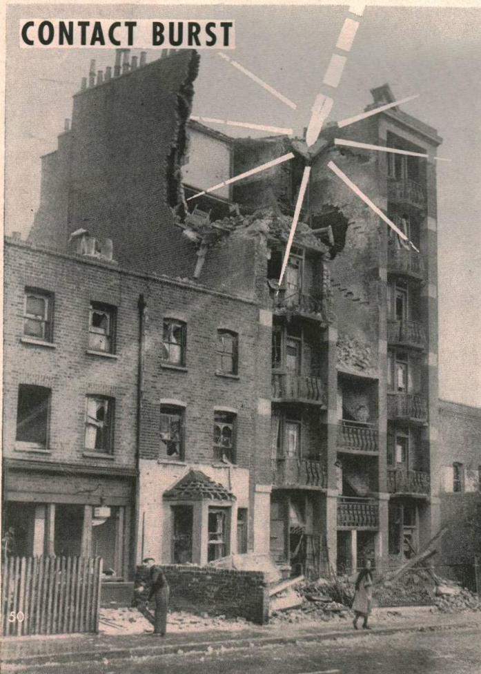
WITH FUSE SET FOR CONTACT, BOMB EXPLODED THE INSTANT IT PENETRATED ROOF
