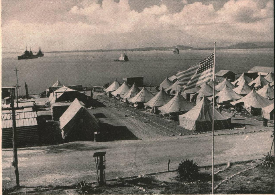
Temporary Marine barracks are built on the shores of Guantánamo Bay. Instead of small two-to-three-man tents previously used in the field, the Marines use py-
