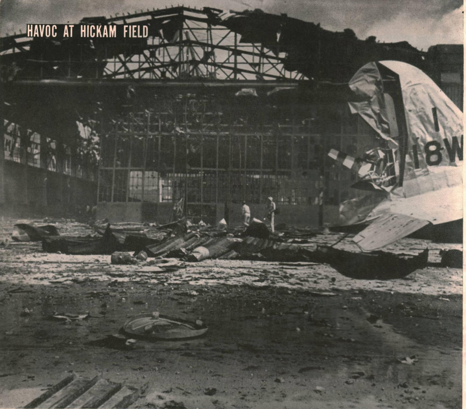
A SHATTERED SKELETON IS ALL THAT REMAINS OF HANGAR NO. 11 AT THE ARMY'S HICKAM FIELD. LITTERING THE FOREGROUND ARE SECTIONS OF ROOF, THE WRECKAGE OF A B-18
