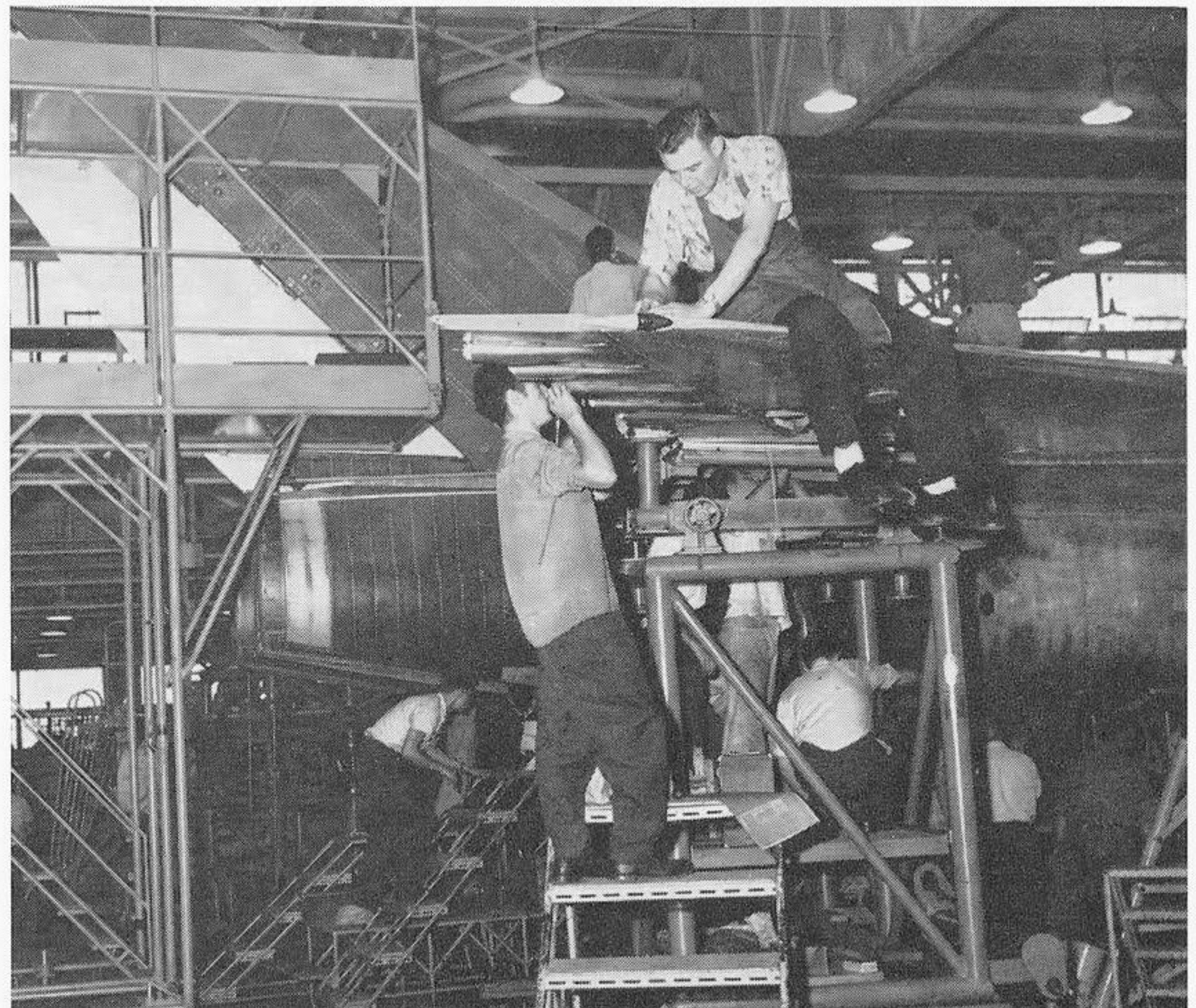
Quality Control inspectors okay each step of the complex Arrow assembly. Here, final adjustments are made to the starboard wingtip by Wally Grandey, left, and Bill Osborn of assembly.
