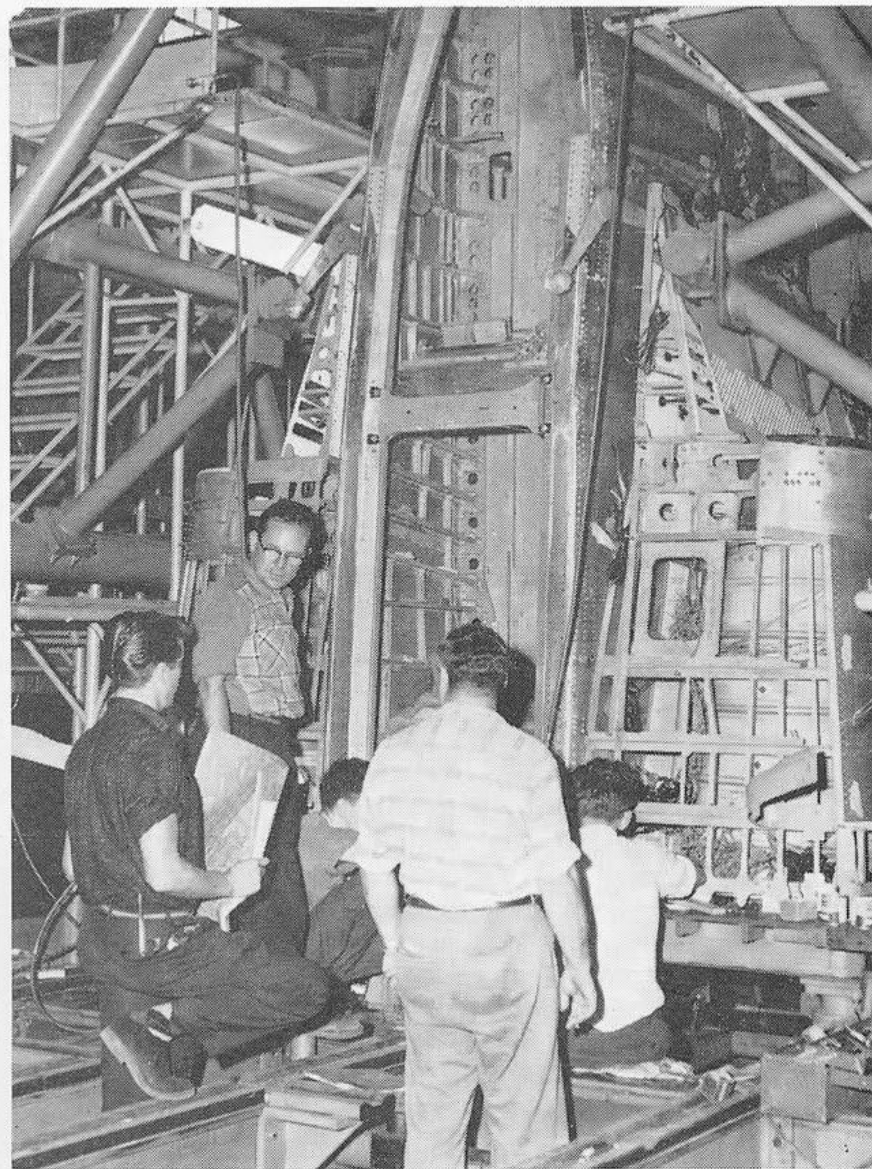
Assembly progress is continually checked against drawings. Here in its jig is the front fuselage section showing both cockpits and engine air intakes.
