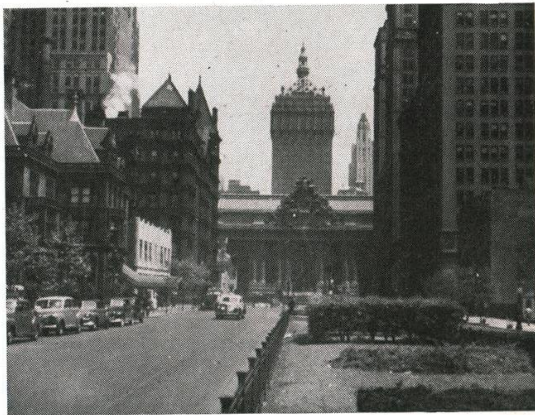
Park Avenue, looking towards Grand Central. 99 Park on extreme right.
