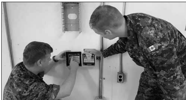
ATIS QL3 students testing their CCTV installation. All Photos Supplied
