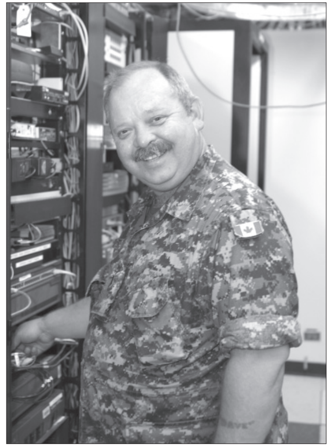
Cpl Dave Hoddinott performing maintenance in a telecom room.
