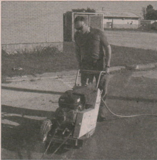
Cpl Starman from W TEME cutting the asphalt for removal.
