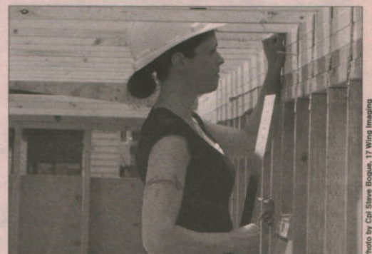
Pte Crystal Brown, AVN technician with 402 Squadron enhances her newly developed skills at the Habitat for Humanity Winnipeg volunteer building site in Transcona on July 30. Pte Brown and 19 other members of 402 Sqn spent a week assisting with the construction of eight shelters for needy families.
