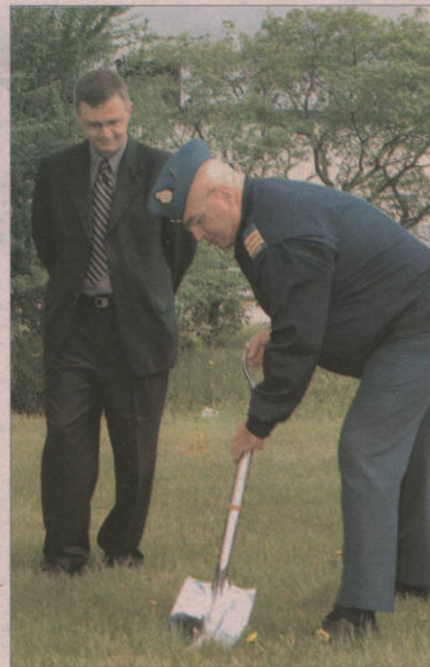
Project manager Lee McCormick watches as Acting Wing Commander LCol Jim Kerr turns the sod as construction is about to begin.
