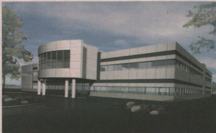
The brand-new Wing Headquarters – expected to look like this – will greet personnel on the Wing immediately past the Whytefold gate.
