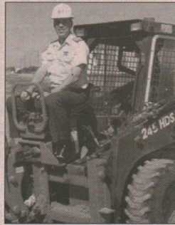
Col Kummel initiates demolition of an obsolete Det Dundurn building while visiting the Detachment.
