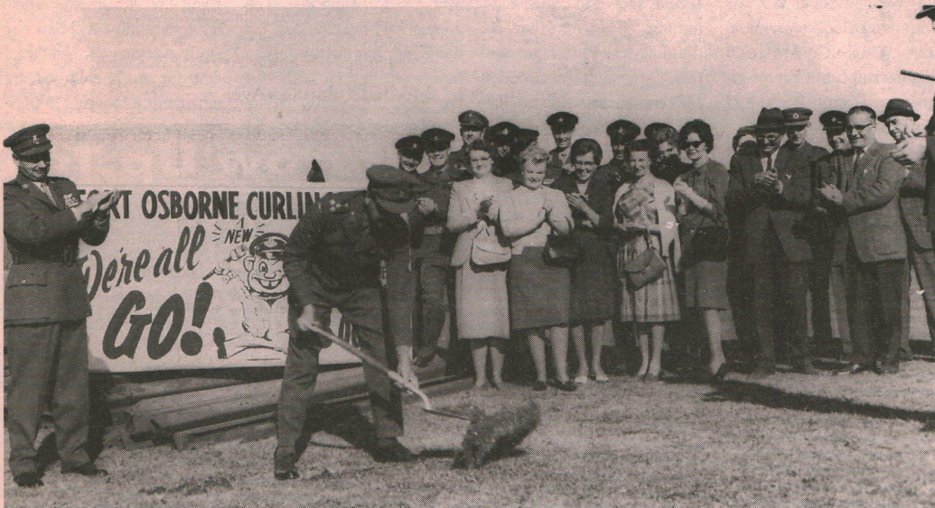
Brigadier General Pangman turns the sod to open construction on the curling club.
