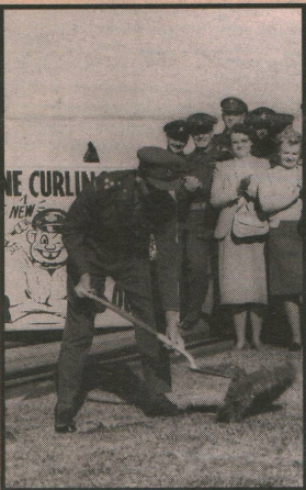
Brigadier General Pangman turns the sod to open construction on the curling club.
