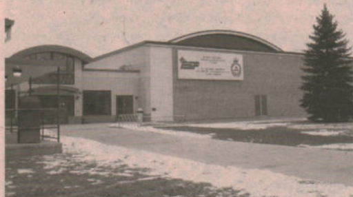
Fitness and Recreation Centre (Bldg 90)
