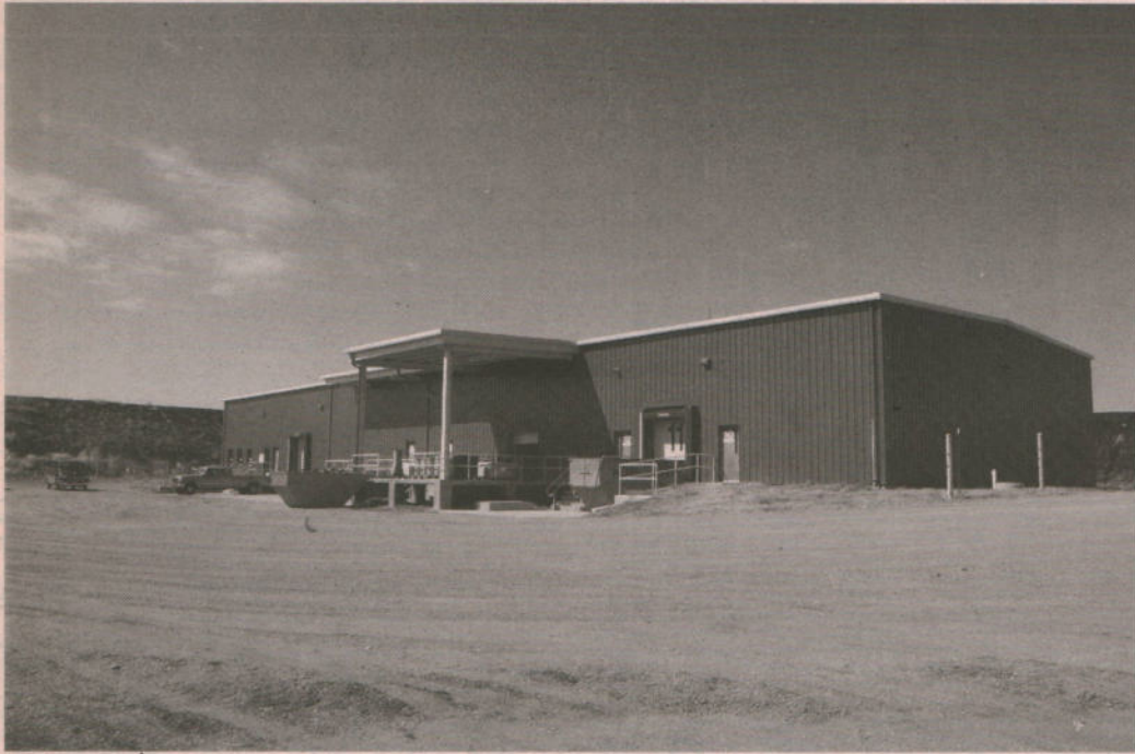
The Ammunition Processing Building at Canadian Forces Ammunition Depot in Dundurn, Saskatchewan.
