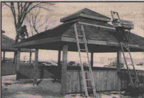
Snow may have fallen, but the patio is in and finishing touches are being made (Dec 99).
