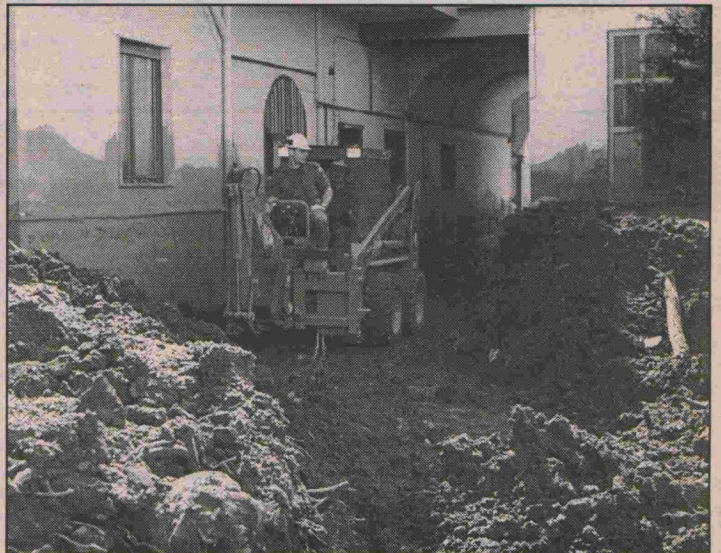
Photo from DND web site.
