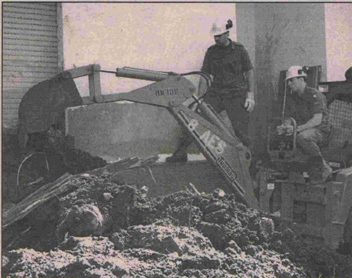
Photo from DND web site.
