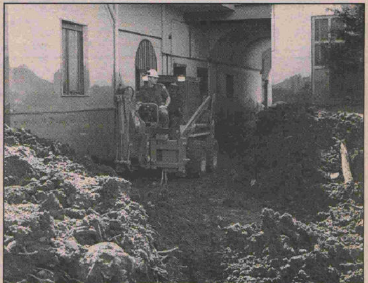
Photo from DND web site.
