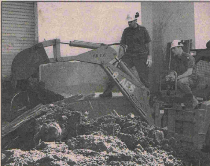
Photo from DND web site.
