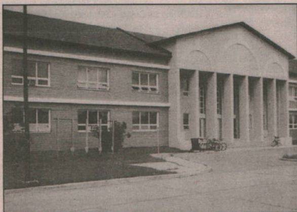
A new facade and siding on Building B-11.
