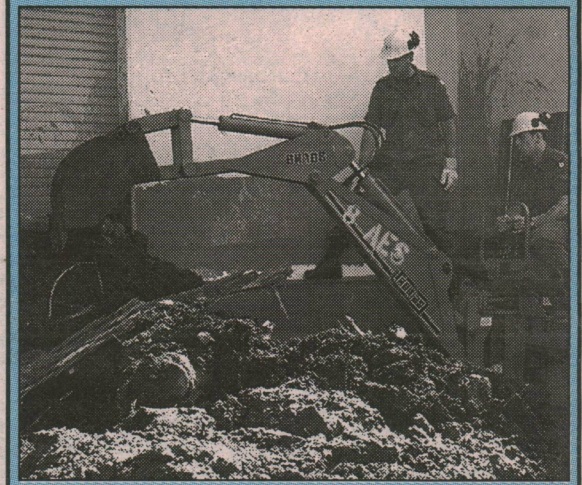
19 May 1998 - MCpl Marty Wilkinson from Kitchener, Ontario and Cpl Pierre Bertrand (backhoe operator) from 17 Wing Transport Sqn, took, carefully, the first Canadian Forces scoop of dirt from the mud slide disaster this morning after spending the night at an Italian Armored Regiment Barracks in Fratte, Italy. The first seven of the ten Bobcats on the ground here in Sarno started working this morning after doing a test of their equipment. The remaining three Bobcats are expected to arrive in Naples around noon today and will start work first thing tomorrow morning. DND photo by Cpl Peter Redden.
