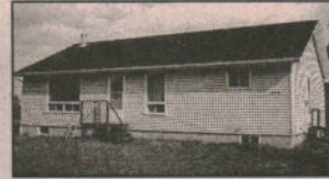
HARVEY, $49,900: Acre with a barn, large bungalow, 30 minutes to Fredericton. Walk-out basement.
