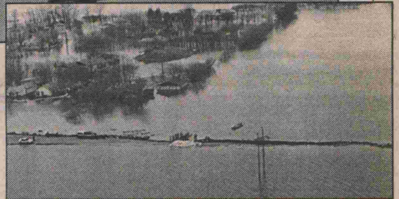
Many roads and highways in Southern Manitoba have all but disintegrated from water erosion, leaving many communities with few access routes.
