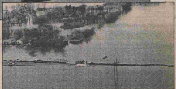
Many roads and highways in Southern Manitoba have all but disintegrated from water erosion, leaving many communities with few access routes.
