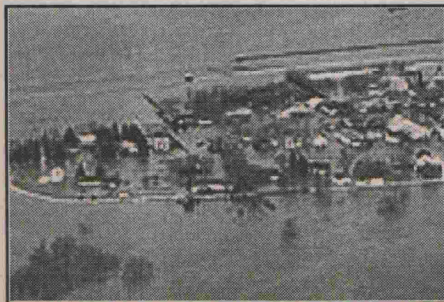
Town of St. Agathe showing the flood breach in the dike. (Seen in the top left area of this photo.) The town flood level reached a height of 2 meters. (Low res., digital image.)
