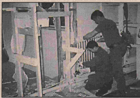
MCpl Steckly and Cpl Fortin during a removal of cast iron radiators from the steam heating system.
