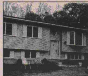
15 MINUTES TO BASE. 3 bedrooms, eat-in kitchen, lower level with recreation room and rear walk-out, separate dining room, excellent water, well located in a treed area. Price $119,900.
