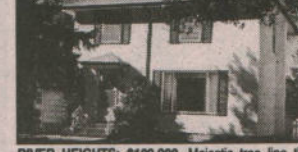
RIVER HEIGHTS: $109,900. Majestic tree line the street of 2 storey homes. Hardwood floors, 3 season room off dining room. Double detached garage. Delightful family home in mature area.
