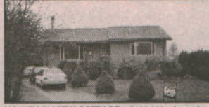
MOUNTAIN VIEW COTTAGE: $130,900. Located on quiet rural side street of North Courtenay, this cozy character cottage offers spectacular views across private back yard. Birch cabinets and fireplace add to the hominess as does the bay windows.
