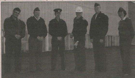
Then, old building 90 - Oct 93 WComd Proulx turning the sod.
