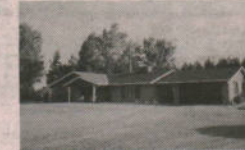
SPACIOUS AND GORGEOUS RANCHER: $179,900. Over 2,600 sq. ft. of living space, 4 bedrooms, 4 pc. and 3 pc. baths, huge kitchen with centre island, cultured floor, fireplace. TR-527.
