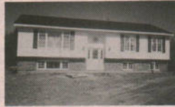
LOT 92, 19 COLLINS ST. $138,900: Cromocot area. New subdivision, newly constructed 3 bedroom split entry home. Eat-in kitchen with built-in appliances, separate dining room. 1 acre lot. Private backyard.
