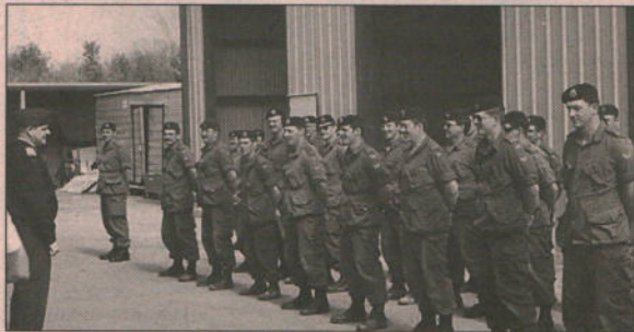
Col K. Penney addressing the Canadian Construction Engineering Squadron in front of the 3 Bay storage building constructed for the 153 CES.
