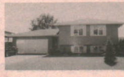
GRENADE VILLAGE: $187,500. Ranch style split entry bung. Upgraded. 3+2 bedrooms. Large family room w/heater FP, walkout to inground pool. New soffits & fascia. 5 min. to base.
