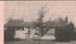
SOUTH WOOD PARK: $90's. Only 10 minutes to base & all the convenience of Fredericton shopping. Lovely 3+2 bedroom home with walk-out basement, finished with 2 baths, family room, wood stove.
