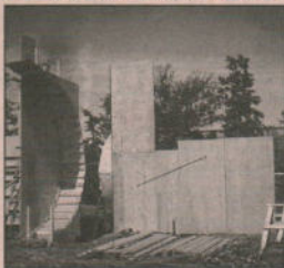
Work on the pedestal for the CF 101 is nearing completion.
