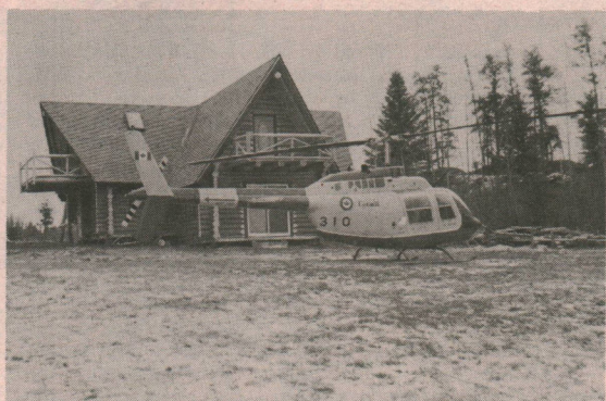
Cabin after clean-up.
