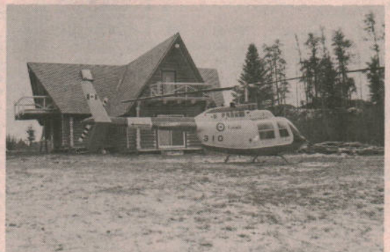
Cabin after clean-up.
