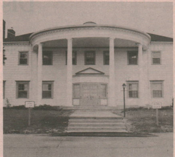
Front view of the CFB Cornwallis Officers' Mess.
