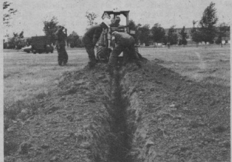
CommSqn super mechanical gopher from Krypton cutting trench from AirCom HQ to Base HQ to lay new 600 pair cable which will replace water-soaked 200 pair cable. (BASE PHOTO)
