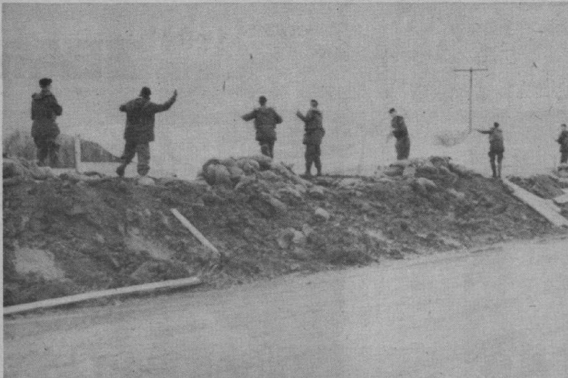
Troops of 2PPCLI lay protective sheeting over a dike to prevent erosion.(PHOTO BY CAPT J. CASEY)
