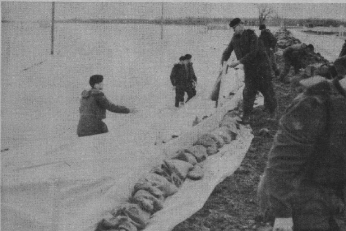
Protective sheeting is "anchored" to a dike using sandbags as weights. (PHOTO BY CAPT J. CASEY)
