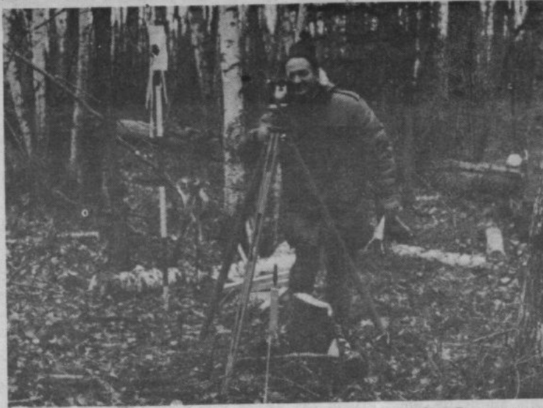
Walt Gidyk of Base CE is shown surveying the Campground Roadway
