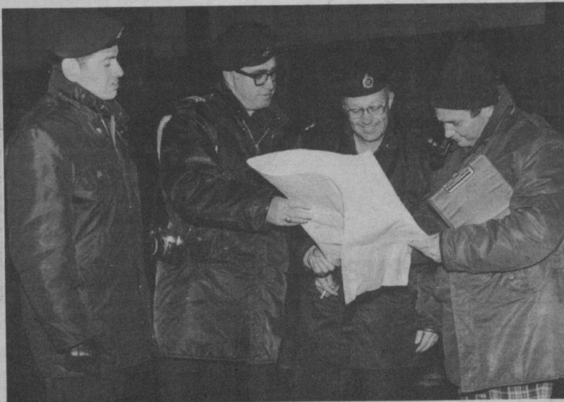
Mr. Gidyk of the CE Section is shown explaining a feature of the accommodation proposal to the BTSO, LCOL. McNeil, and CAPT. Waddell of Base Supply. CWO. Pilote of BML looks on (BASE PHOTO)
