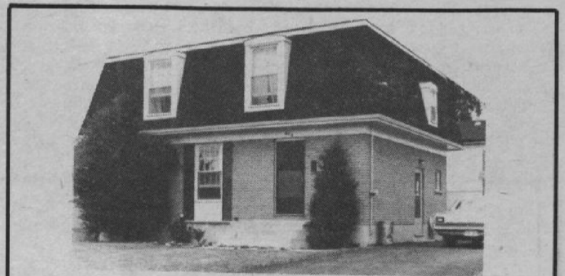
626 Bridge St. E. Belleville
