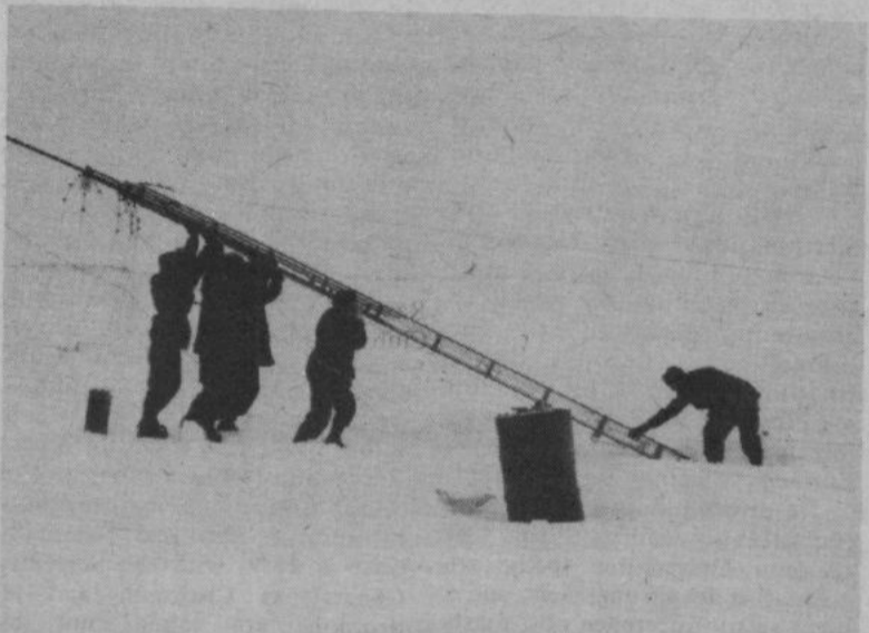
Despite the snow-covered solid ground, the crew successfully erected the 180-pound steel mast to support the Multi-Band Transmit Antenna.
