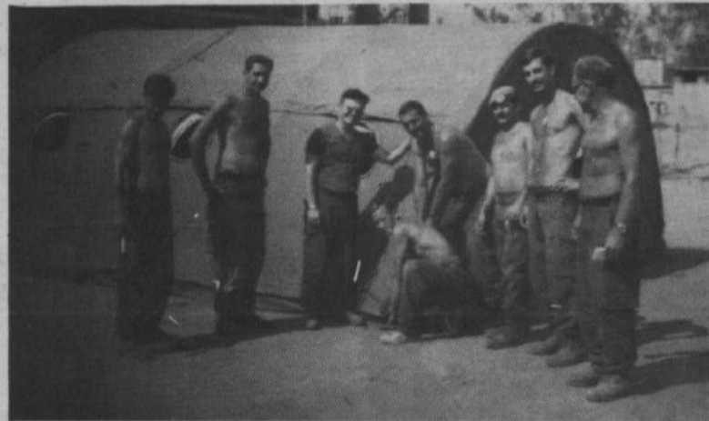
Members of the 116 ATU advance party in Ismailia stand before one of the Polish tents they erected. Similar tents will be used to house many Canadians until hard accommodation is available.
