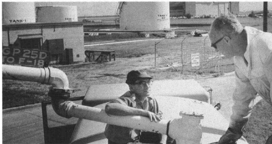
Sgt. Tom Jackson and Cpl. John Klassen swing the Loading Arm into position to top up one of the five fueling Tenders needed to completely refuel a 707. Photo by Hoover
