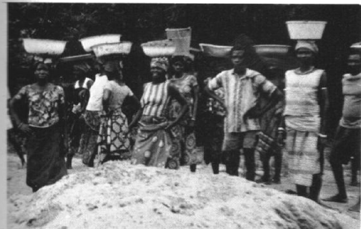
SAND, scraped from the bed of the Volta River is transported to the school site by the Villagers for use in cement construction blocks.
