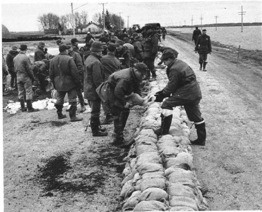
PREVENTIVE MEASURE. Members of 3RCHA prepare a dike east of Carman where the swollen Boyne River threatened more flooding.
