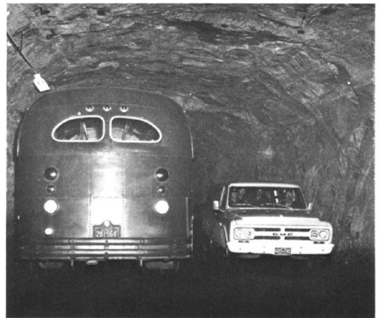
CLOSE FIT — Deep beneath the Laurentian Mountain Range, a vehicle pulls into a passing slot to yield the right of way to a shuttle bus. The access cavern leads to the subterranean NORAD defense fortress at Canadian Forces Base North Bay, Ontario. The professional miners constantly check the cavern to assure safety for men and equipment. (NNS)
