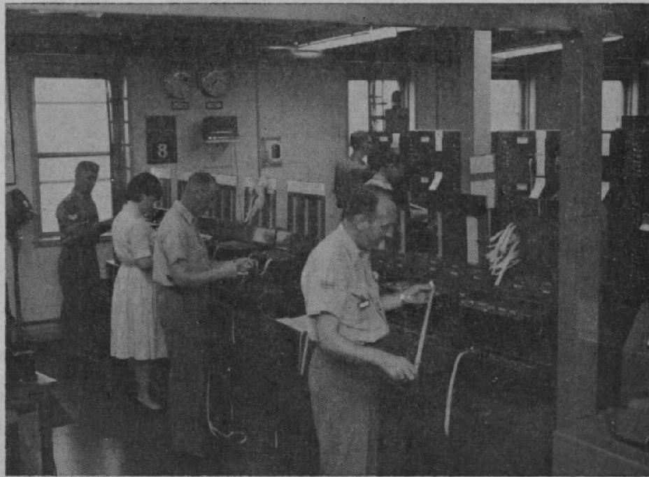
3CU Tape Relay Centre.
