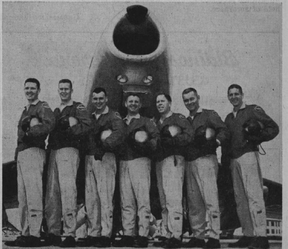
Persons who pride themselves in aircraft identification can be expected to have difficulty with this Air Defence Command plane. It's actually a modified Dakota based at RCAF Station Yellowknife. The long extended nose cone houses delicate radar equipment which is an exact duplicate of that found in the CF-104 Starfighter. The radar is used for low level navigation of the supersonic 1,400 mile-an-hour Starfighter. Initial pilot training is carried out in this modified Dakota that flies along at low level at a comfortable 140 miles an hour.
