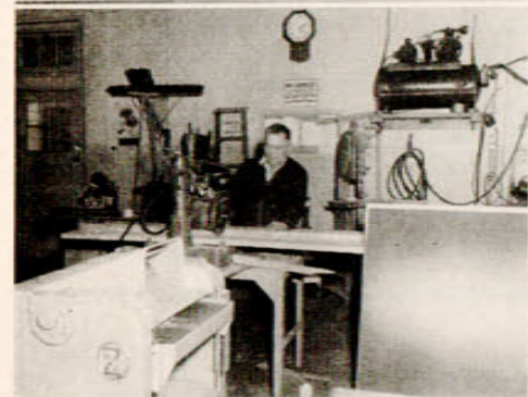
Mr. W. Trescor, carpenter Shop Foreman, prepares to operate radial saw in carpentry shop.
