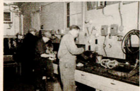
Electrical shop: Left to right—Mr. V. W. Wicklund, Mr. G. Dickson, electrician, and Mr. G. Harrop. Mr. Harrop is assembling explosion proof light fixtures used in fuel tender bays, etc.
