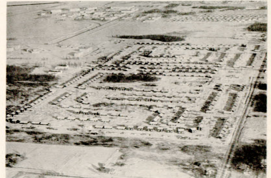
The new Stn. Winnipeg married quarters are shown in a recent aerial photo. More than 150 families are already occupying the quarters being constructed by the Metropolitan Construction Co. Ltd.
