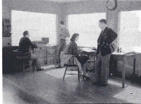
The Control Tower
