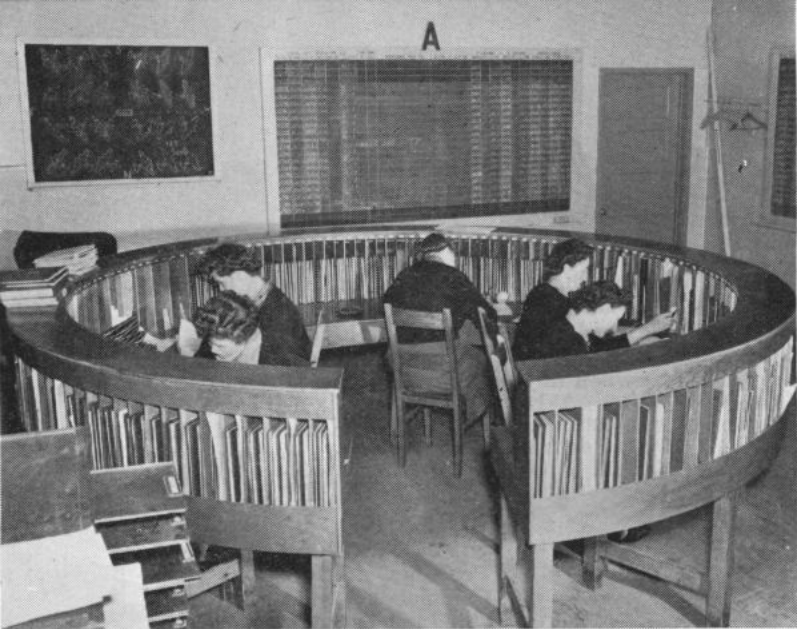
MAINTENANCE CONTROL ROOM
